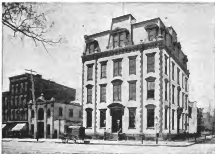
320 PRECINCT (MOUNTED) POLICE STATION, AMSTERDAM AVENUE AND WEST 152 d STREET.
